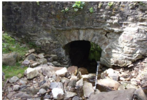
Single Span Stone Arch Over Old Horseshoe Pike
