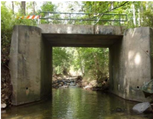
East Box Beam Bridge at Bondsville Mill Park
